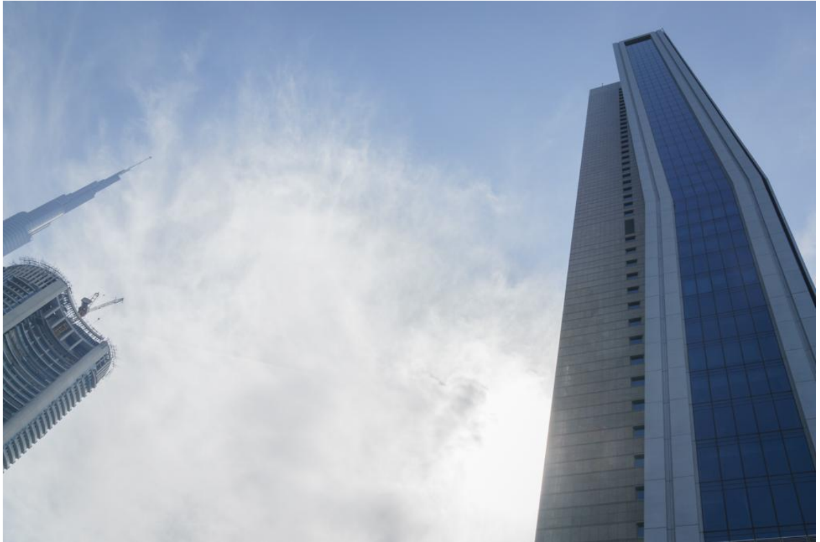
Burj Khalifa, Baustelle, Burj Gate
